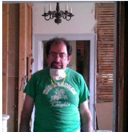
Left, ruined debris from Hurricane Irene flooding is set by the curb in Schoharie, NY. First Pres member Alan Northrup grew up in Schoharie and helped clean up the mess. Behind him can be seen some of the stripped walls.
